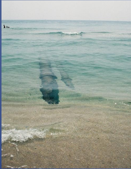
Illegal A/C drainage pipes
